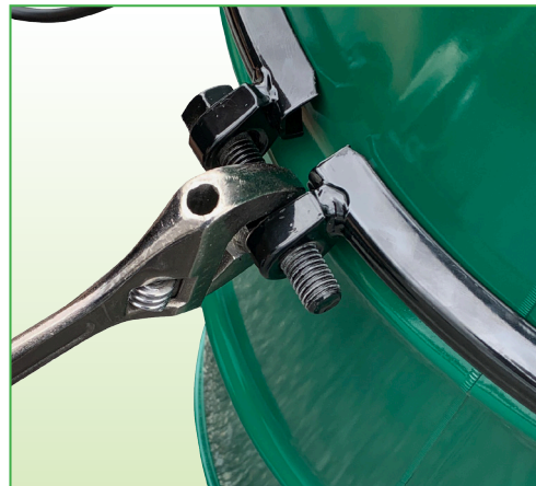
6 Adjust both bolts making sure not to over-tighten and damage the drum.
